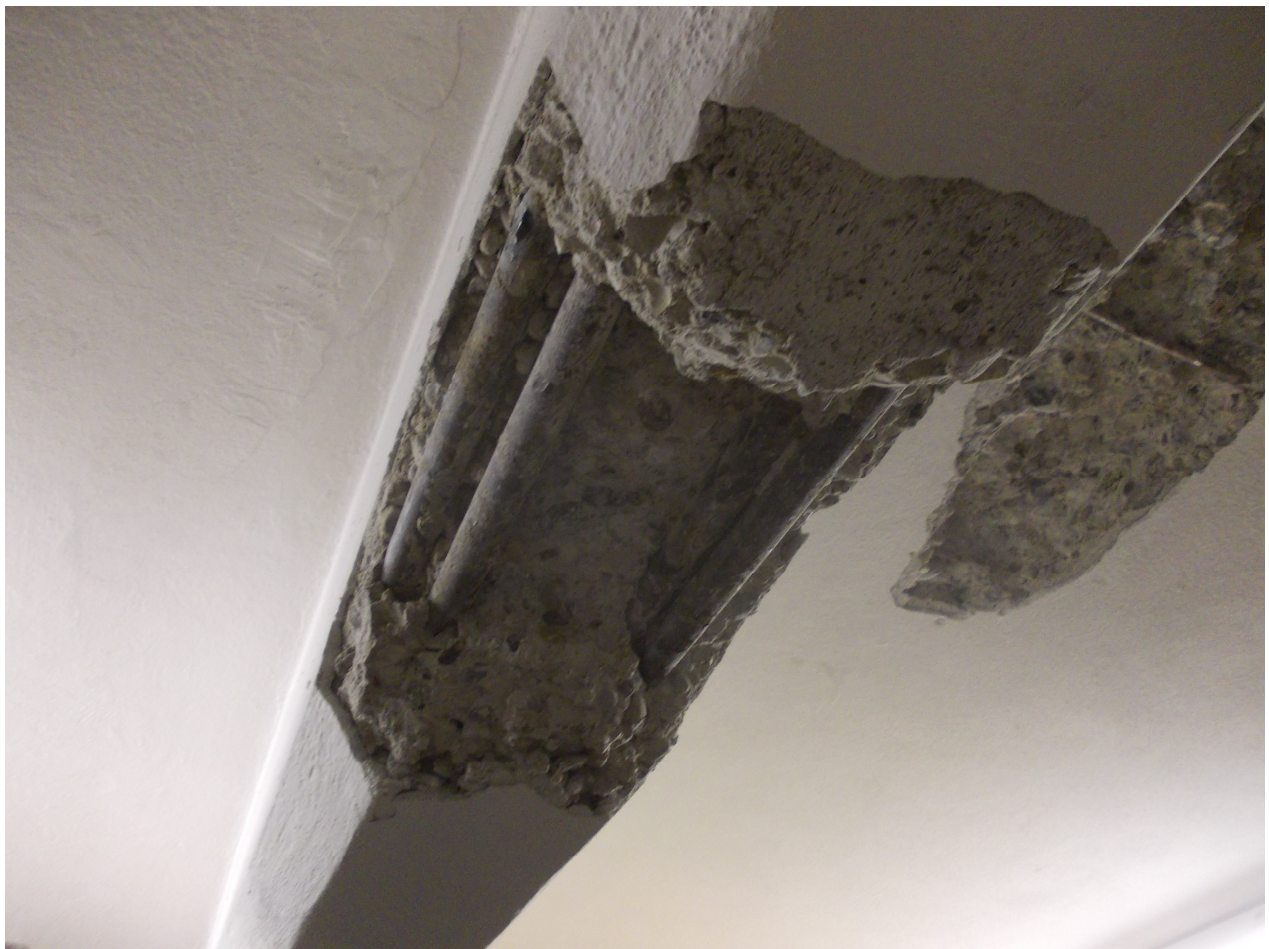
sondaggio 14 – trave in c.a.
