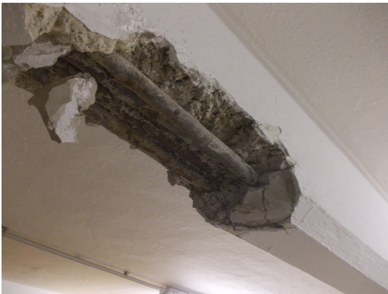
sondaggio 11 – trave in c.a.
